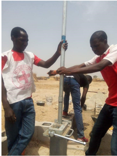
NRCS volunteers supporting in the construction of a water point
